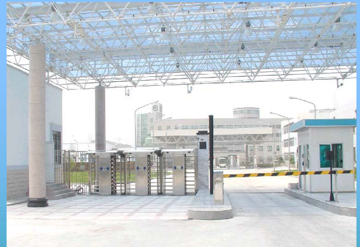
Access control system Qinshan Nuclear Power Station
